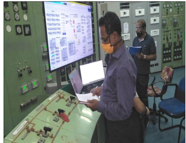
Measurement of Power at Control Room of Chiplima HEP
