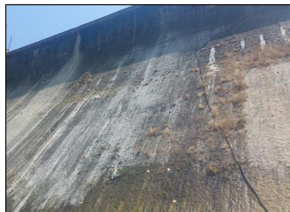
Wire-mesh and Shotcreting on U/s face of the Dam and view of downstream face of the dam at Pre and Post treatment stage showing reduction in seepage.
