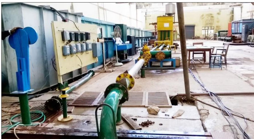
Pump test circuit -piping and Volumetric Tank
