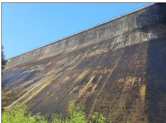
Wire-mesh and Shotcreting on U/s face of the Dam and view of downstream face of the dam at Pre and Post treatment stage showing reduction in seepage.
