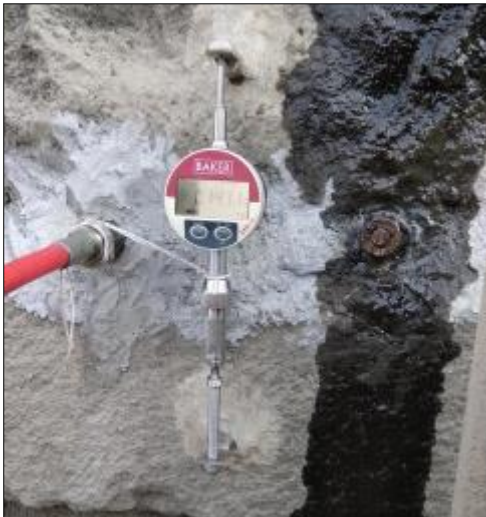
Photo 1. Flat Jack test in progress at Walwan dam
