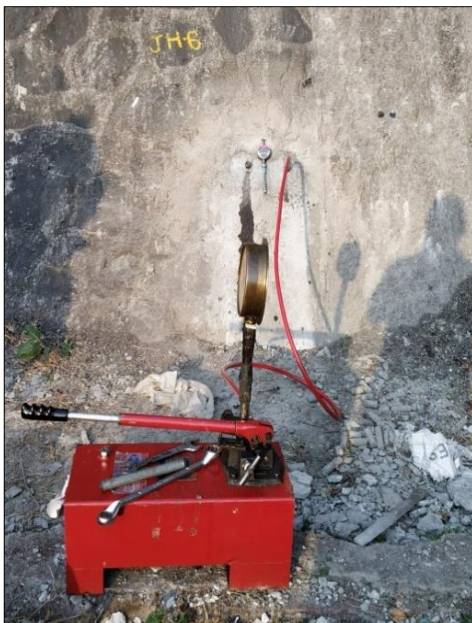
Photo 1. Flat Jack test in progress at Bhatsa dam
