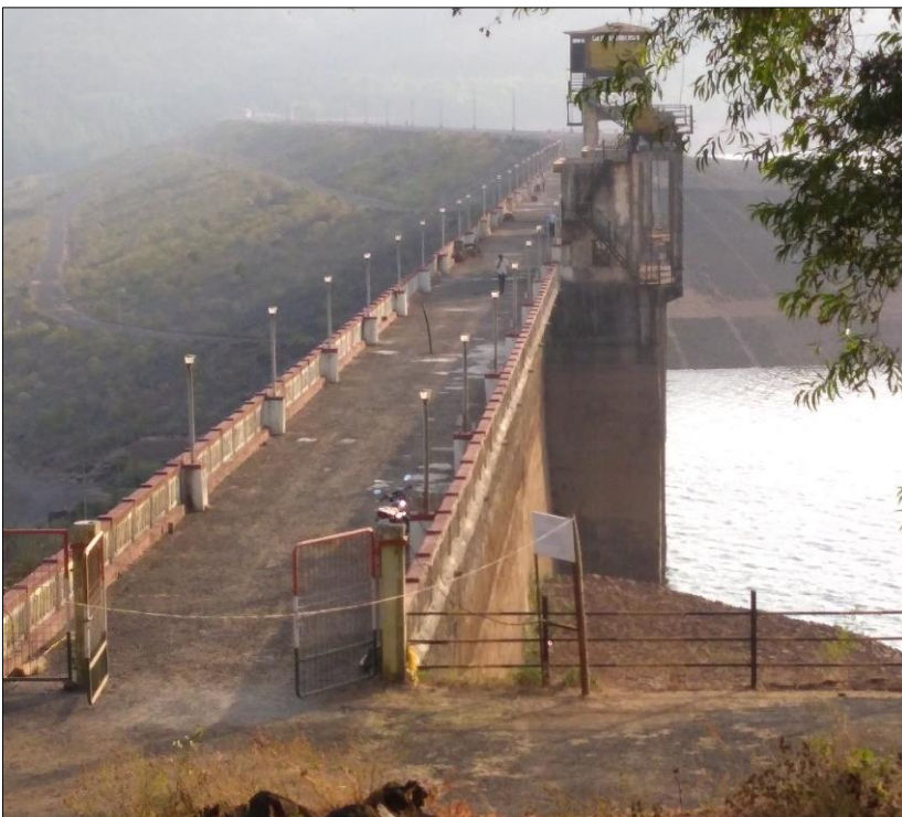
View of Warna Dam Top
